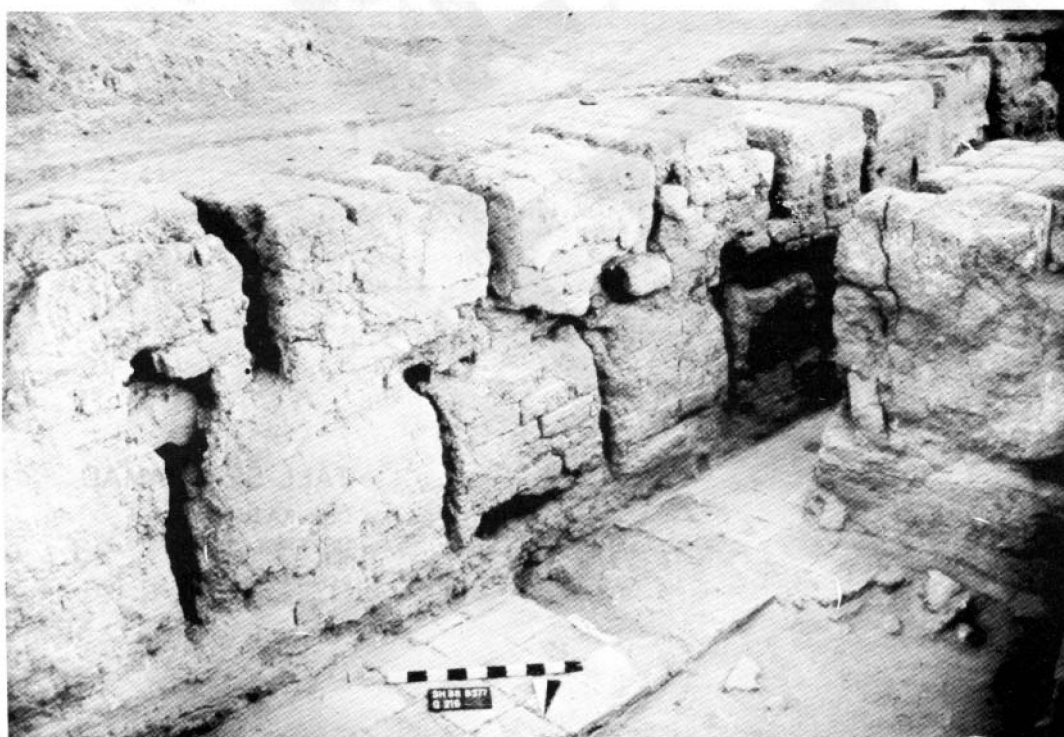
FIG. 11 Room Y and corridor T, from north; east wall (7) with airvents and burned out wooden posts and bearings
